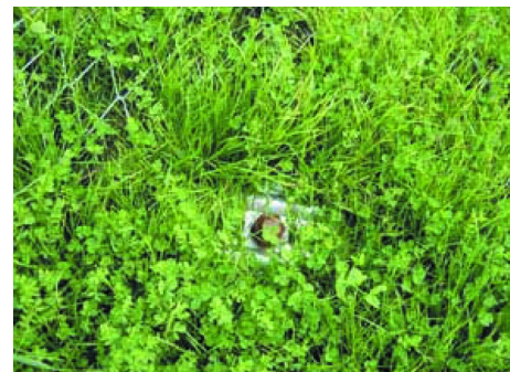
TECCO Mesh and spike plate with Tecmat 400 and greening
