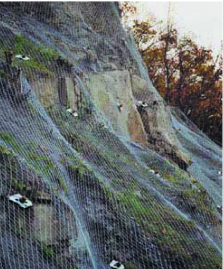
Adaptability of the flexible high-tensile steel wire mesh to the slope surface is illustrated
