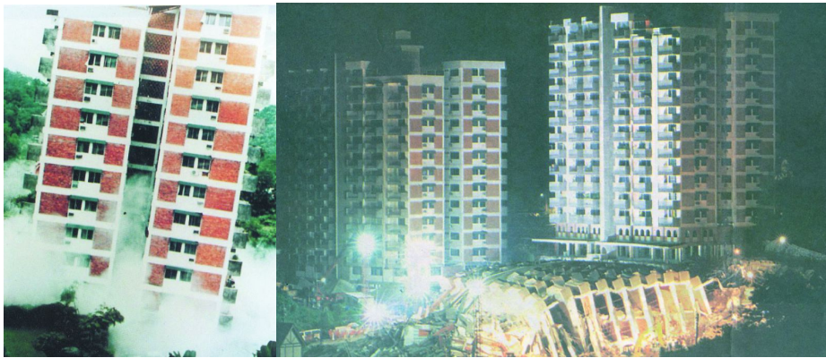
Block 1 of Highland Towers at Taman Hillview which collapsed on 11 December 1993
