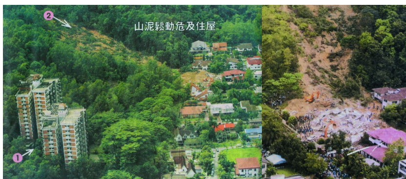
Bungalow destroyed by landslide at Taman Hillview on 20 November 2002
