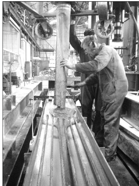
Figure 2: Pouring of fresh SFR-RPC in the girder steel forms
