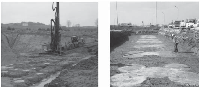
Figure 16: DSM works / exposed columns before placement of a lean concrete layer
