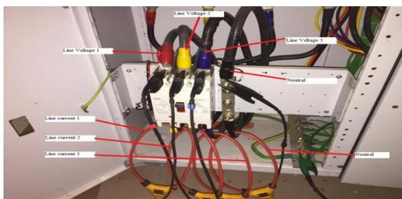
**Figure 2:Fluke 434 connection for measurement**
