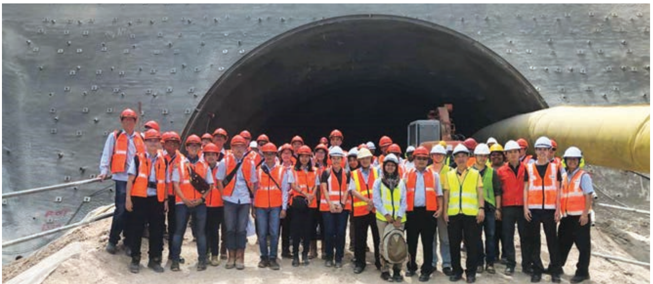
Group photo in front of the V207 tunnel worksite
