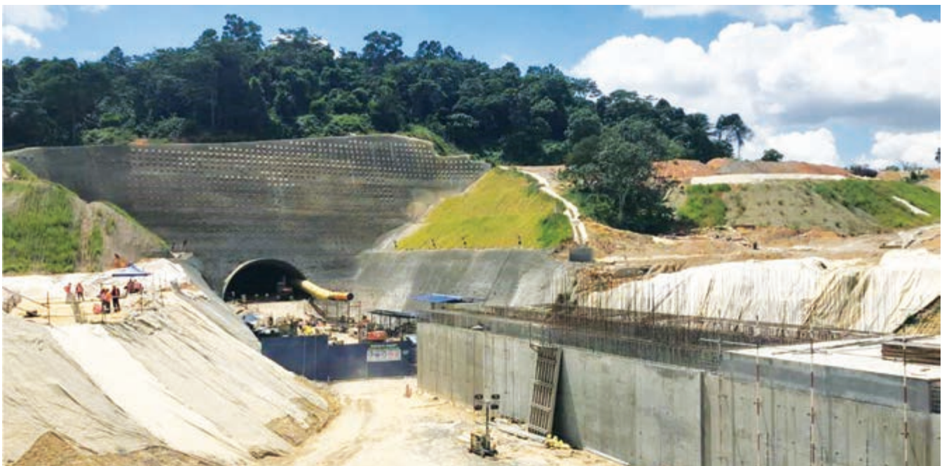
View of the V207 tunnel site in Taman Universiti
