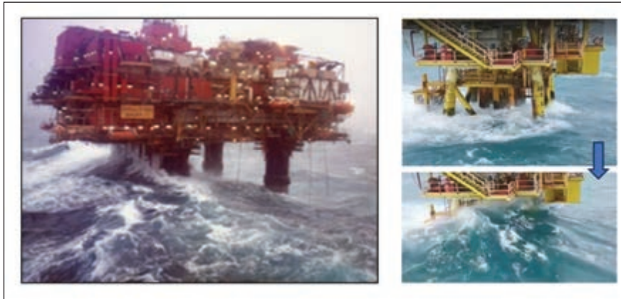
Figure 2: Actual photo of WID loading scenario
