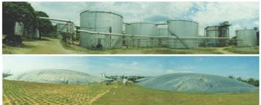
*Palm Oil Mill Effluent (POME) biogas capturing plant*
