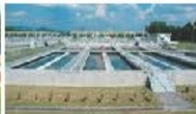
Construction and refurbishment of sewage treatment plants
