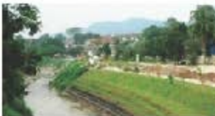
River bank stabilisation and beautification
