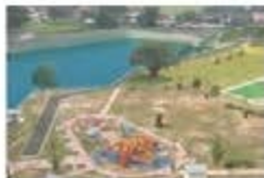
Construction of detention ponds to trap sediments
