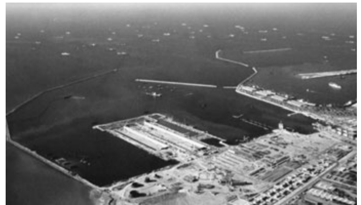
Figure 5: Dubai Dry Dock under construction
