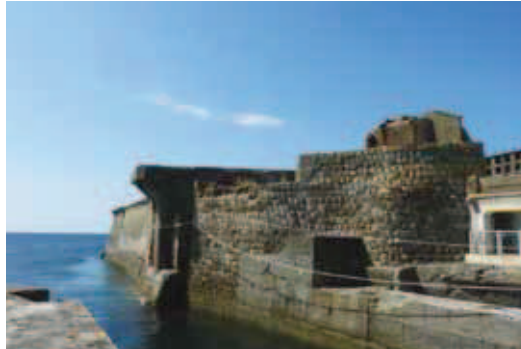
The reinforced concrete wall
