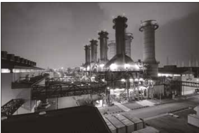
Picture 12: Paka Power Station
