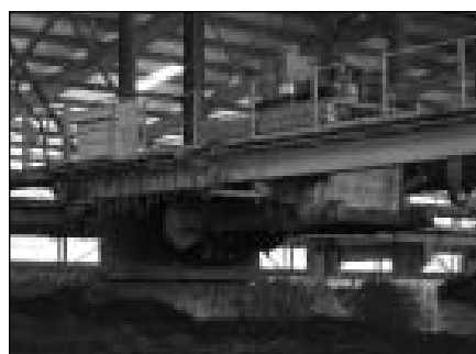
Plate 1: Gantry turner to mix compost materials
