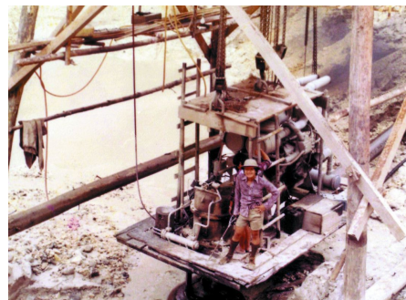
Figure 8: The author with a huge gravel pump which was powered by a 620hp of Cummins engine. Note the size of the engine
