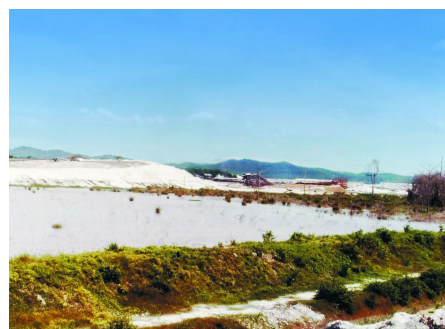
Figure 11: Tailings dump – tailings are stored in impounded dams
