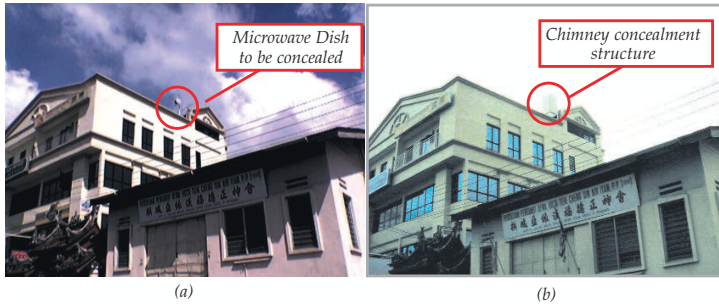
Figure 4: A chimney concealment structure is enclosing a microwave dish (a) before and (b) after concealment
