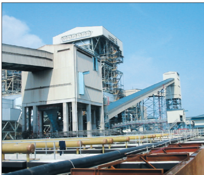
Transfer Tower and Conveyor Belts
