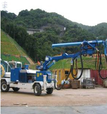
Figures 4 & 5: Applications of Wet Mix Shotcrete
