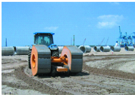
Figure 2: HIEDYC compaction at Westport Container 4 (courtesy of Infratek)
