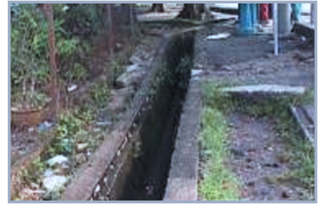
House A with Open Concrete Drainage System
