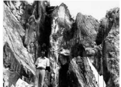
Figure 3: Limestone bedrock arch showing large solution cavity or channel
