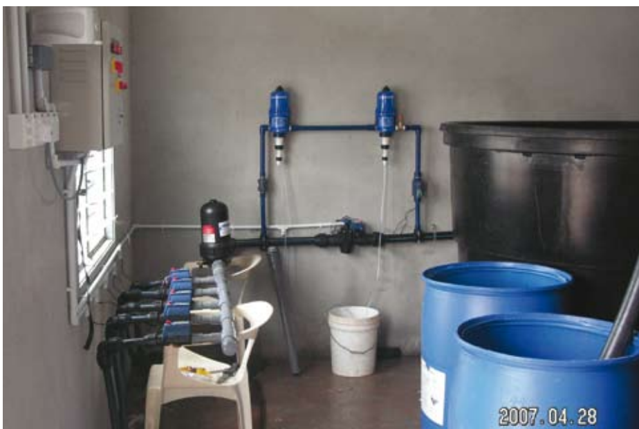
A fully automatic fertigation system using timer, electric operated valves and the liquid fertiliser water powered dispenser
