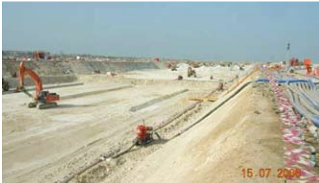
Plate 1: Two levels of well points employed for the dry excavated site
