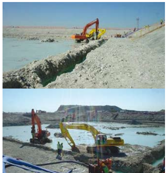
Plate 3: Trench and sump for dewatering system
