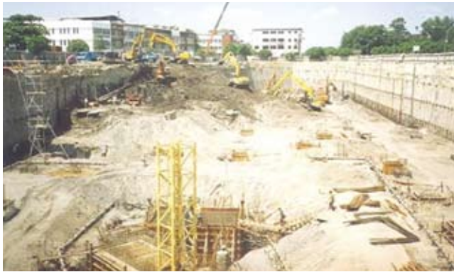
Plate 2: Well points + diaphragm wall for groundwater control
