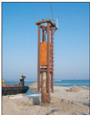
A steel pile being tested using the PDA method
