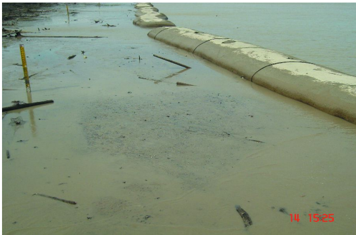
Figure 4: Substrate build-up behind the breakwaters
