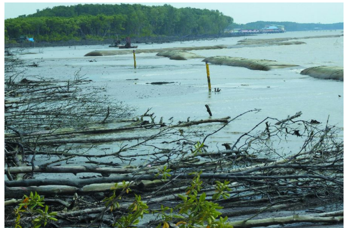
Figure 5: Breakwaters at Tanjung Piai, Johor
