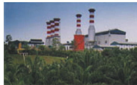
Figure 5: View of Serdang Power Station
