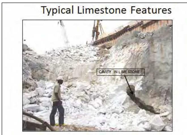
Photo 3: Excavations in Limestone at Velocity Site
