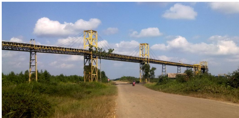
Figure 2.4: Example of Coal Conveyor in Indonesia (Joppe, 2011)
