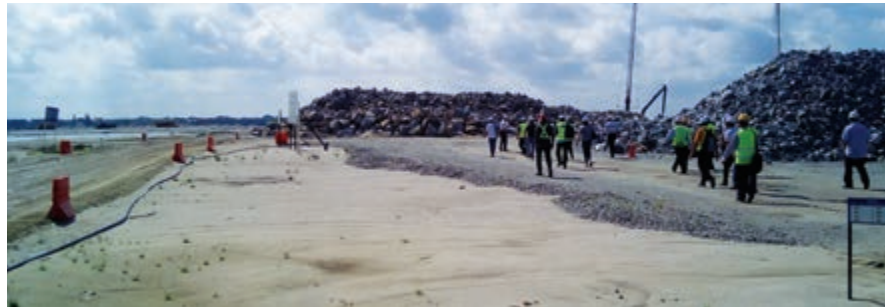
Revetment Rock Stockpile
