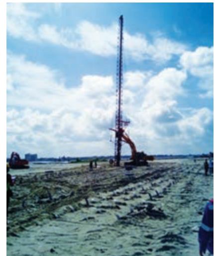
Island 1: Vertical Drain Installation
