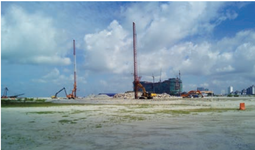
Island 1: Ground Improvement
