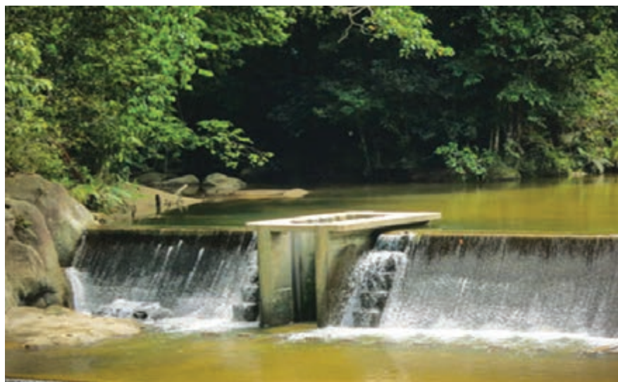
Small hydro-electric is a very matured technology that has great potential to be further developed in Malaysia
