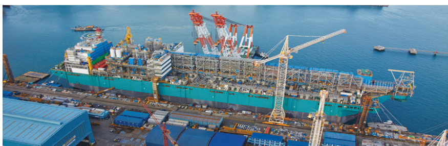
Figure 1: PFLNG1 Construction Aerial View
