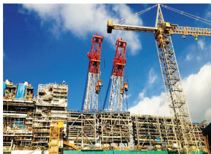
Figure 3: Lifting of the last pipe rack module
