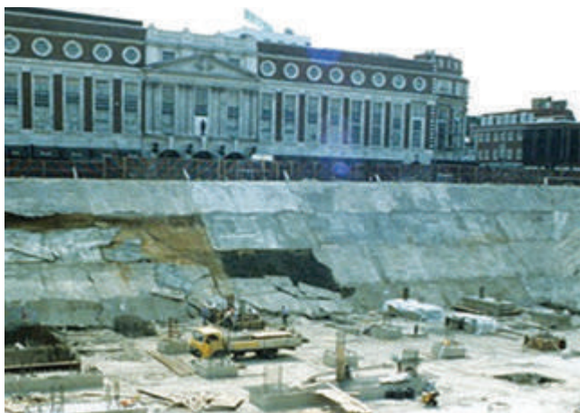
Figure 1: Open-Cut Basement Construction
