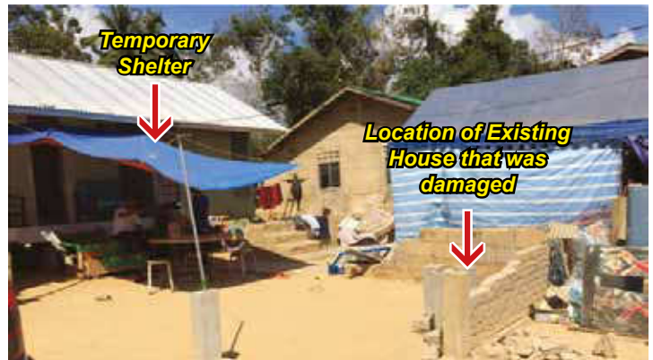
Temporary Shelter for flood victim whose house was destroyed
