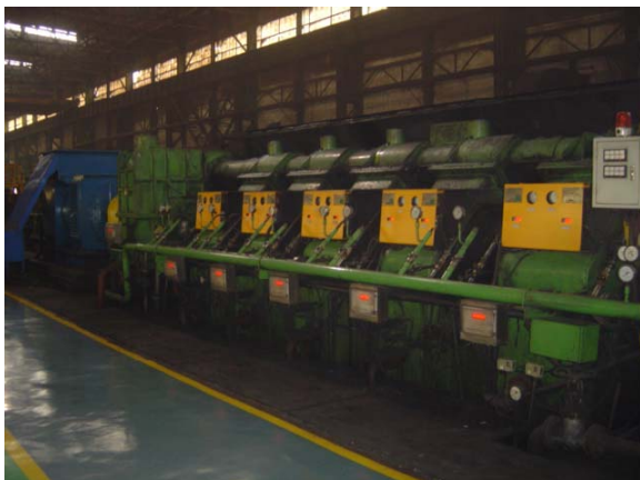
Fig. 1. Anshan Steel and Iron Group wire plant finishing mills.
