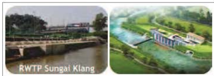
KI 7: River Water Treatment Plant (RWTP)
