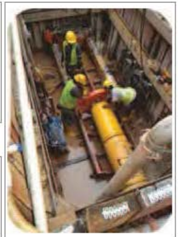
KI 1 & 2: Pipe Jacking for upgrading sewerage
