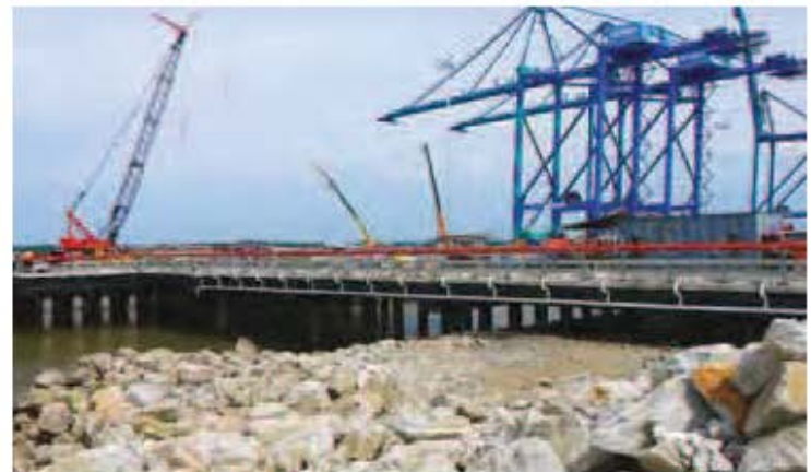
Figure 1: Construction of Bridge25 using UHPdC beams
