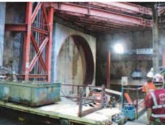
Thrust block in front of launching shaft at MTR tunnel
