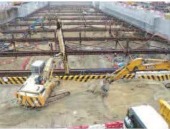
Temporary works for cut and cover tunnel at Austin Station
