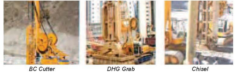
Figure 1: Excavation Techniques in Difficult Ground Condition.
