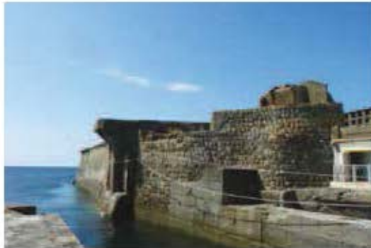
The reinforced concrete wall
