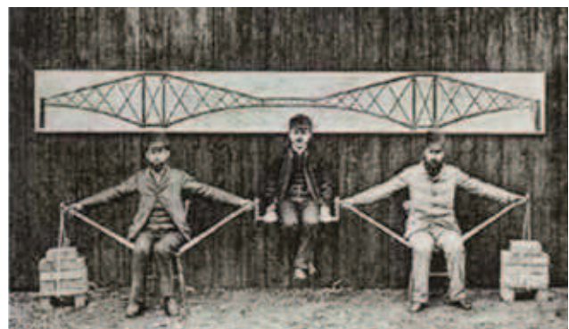
Figure 2: Innovative use of human model to illustrate the design of the Forth Bridge in Scotland
