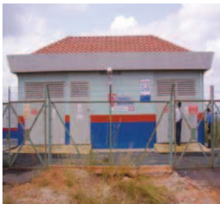
Figure 1: A TNB substation
