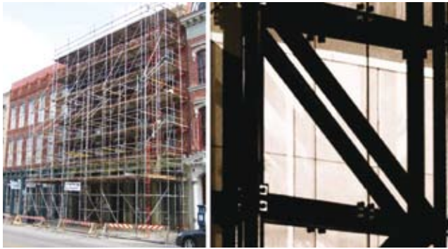
Figure 3: Typical formwork and props in a building facade
