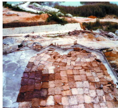
Figure 19: Curing of slabs with moist gunny sacks
