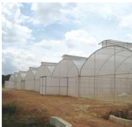
Naturally ventilated insect-screen rain shelter structure
