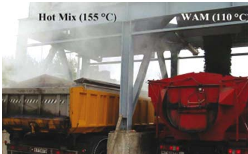
Figure 3: Difference in fume emission between hot-mix asphalt and warm mix asphalt [4]
