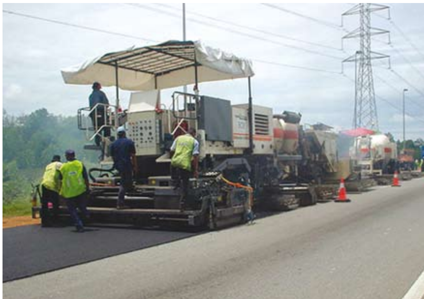
Figure 4: Hot in-situ recycling
