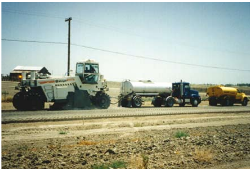
Figure 5: Cold in-situ recycling using foamed bitumen
