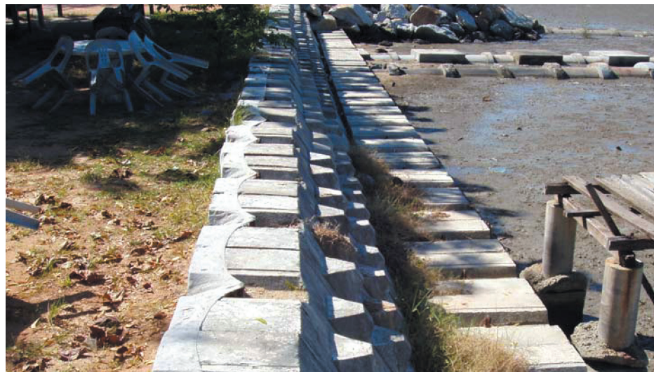
Picture 2: Labuan blocks as sloping “mattresses” (2002)-Taman Robina, Seberang Perai Utara, Pulau Pinang
