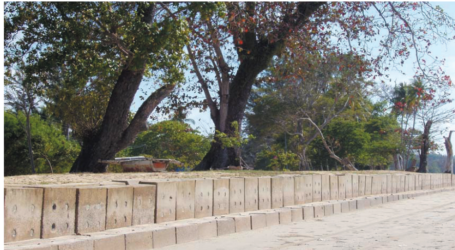
Picture 1: Labuan blocks as vertical cubic blocks (1999)-Pancur Hitam, Labuan
