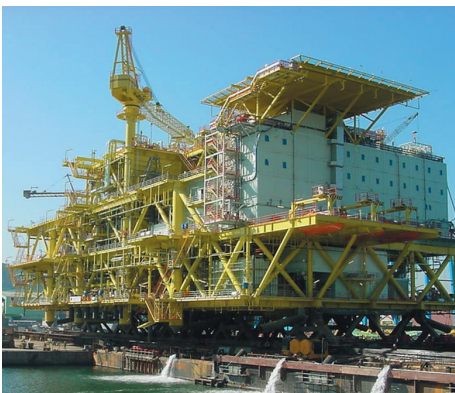
Offshore Platform Project (Topside)
