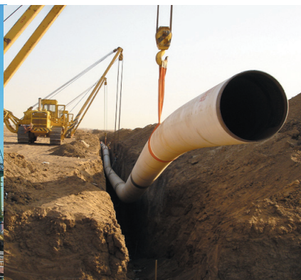
Onshore Pipeline Project
