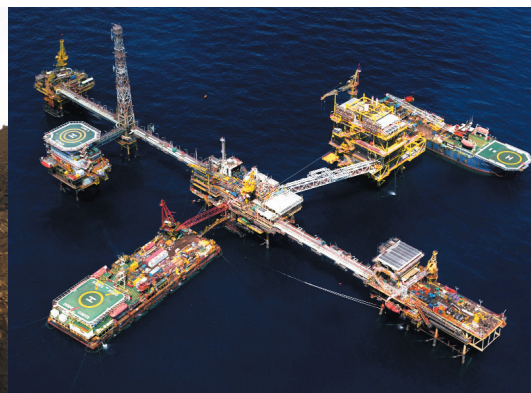
Offshore Platform Complex R&R Project
